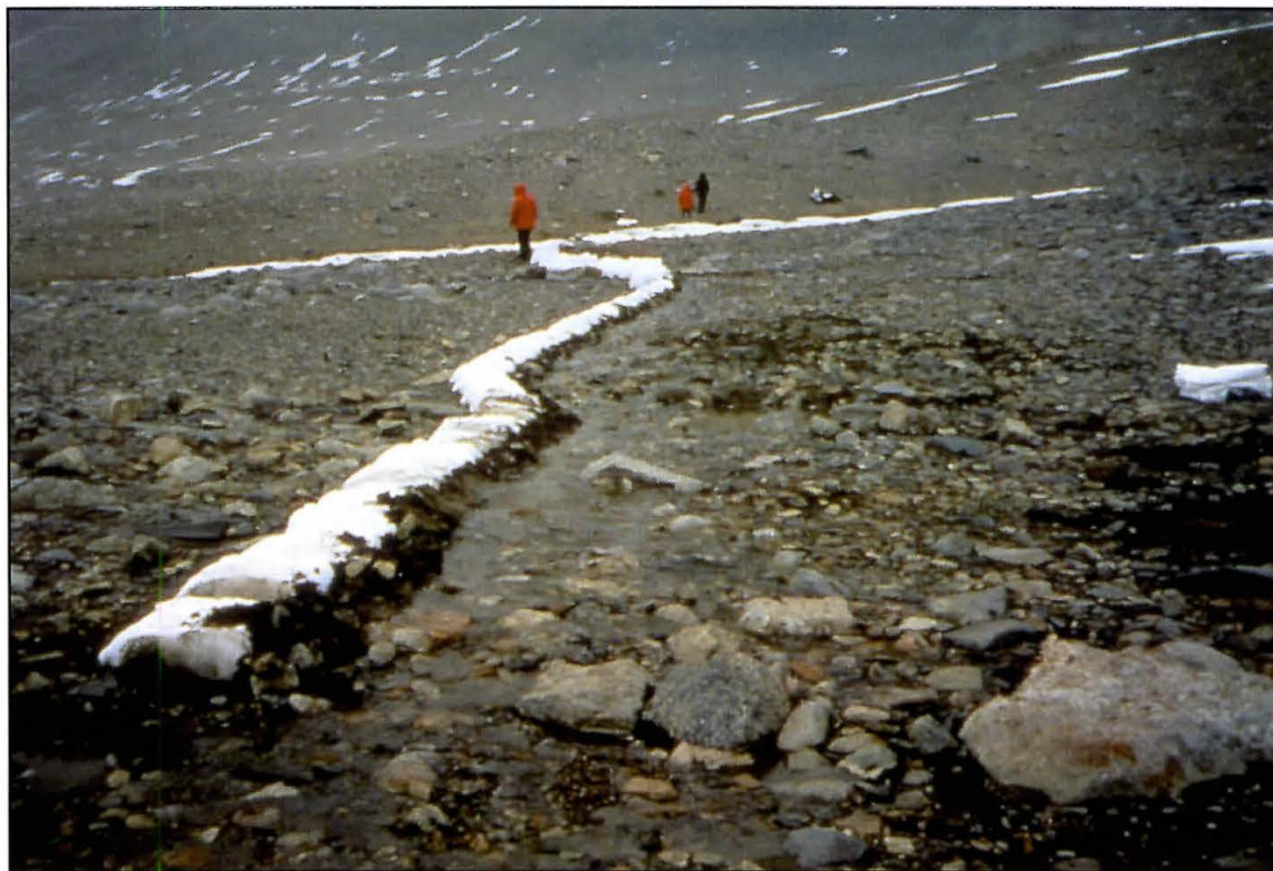
Sandbags are used to direct water into a relic stream channel.
